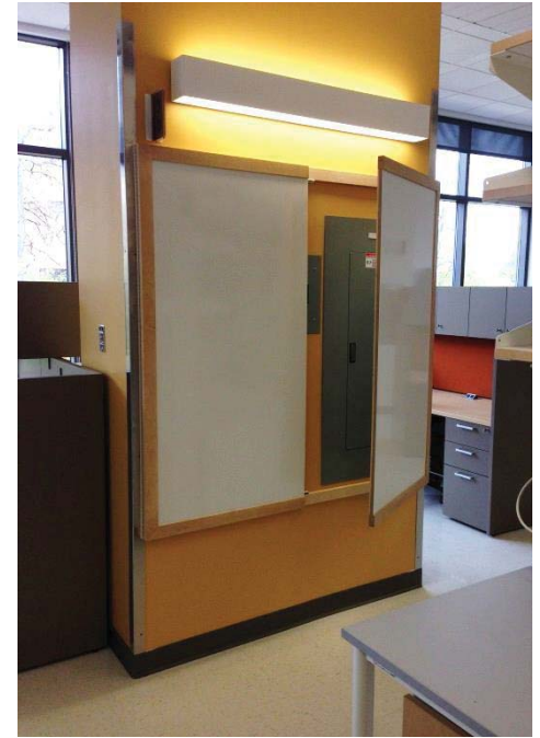
Maximize Discussion Space: Whiteboard Hinged Panels with Electrical and Air Monitoring Control Panels Behind
